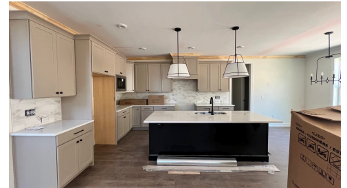
Construction Update May 2026
