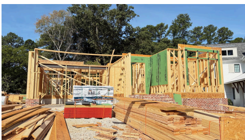
Construction Update - August 2026
