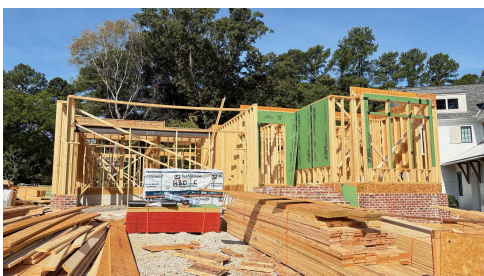
Construction Update - August 2026
