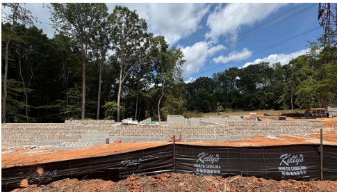
Construction Update - August 2026
