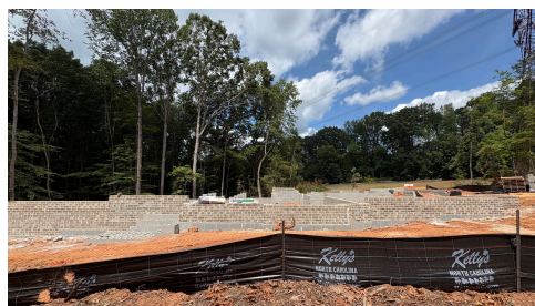
Construction Update - August 2026
