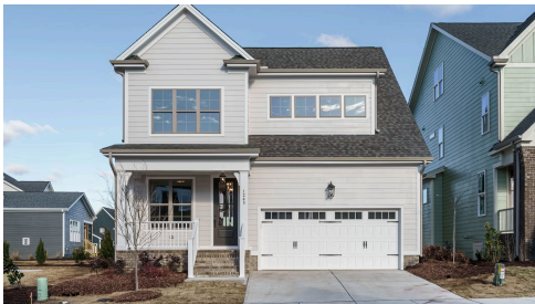
Example of completed Columbia American Farmhouse
