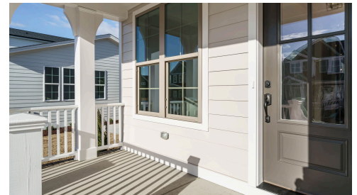
Example of completed Columbia American Farmhouse
