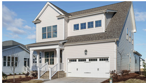
Example of completed Columbia American Farmhouse
