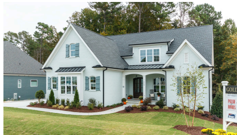
Completed Home Example
