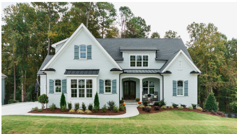
Completed Home Example
